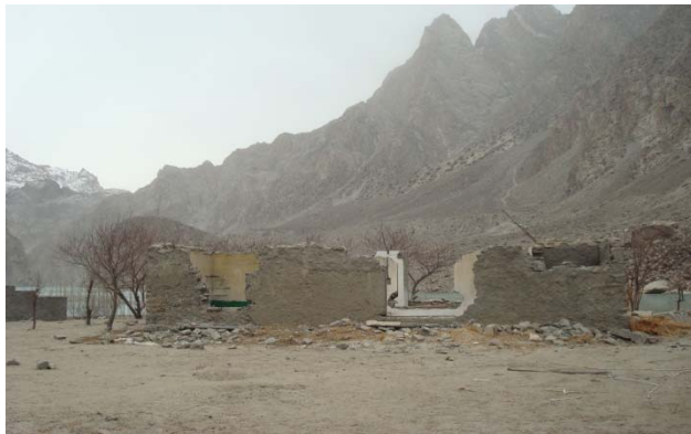
Destroyed Houses at Attabad, Huna Valley
